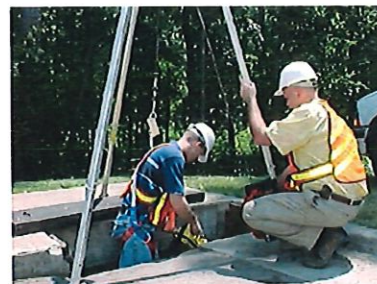
Test for Oxygen levels, flammables and toxic atmospheres before confined space entry
